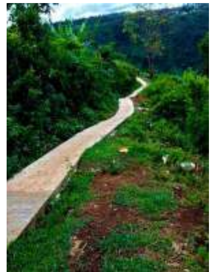
Completed part of the pathway in Barangay Gala, Tudela, Misamis Occidental.
